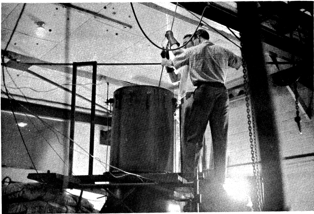
Fig. 6. Lowering the shipping container into tank (rehearsal)
