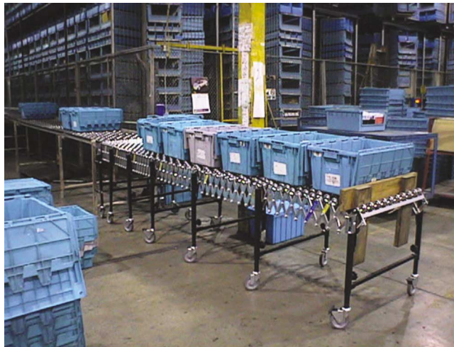
Fig. 12. The new single-level telescoping carousel output conveyor.
