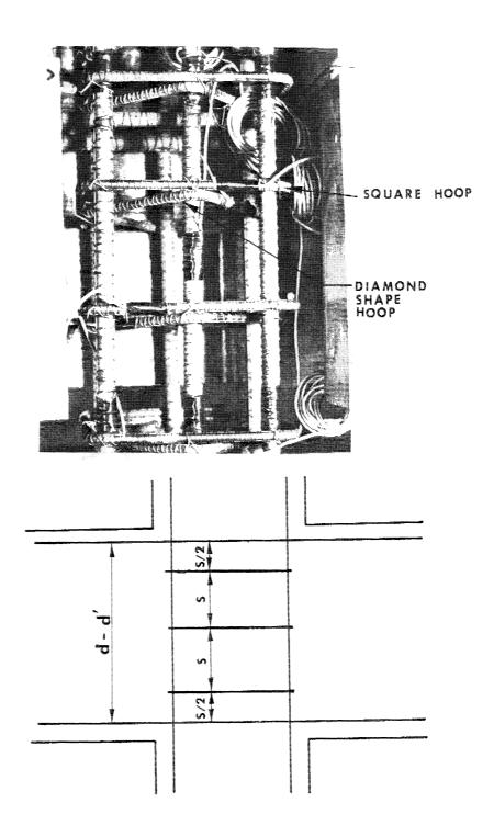
Fig. A.5 Joint Hoop Reinforcement and their Spacing
