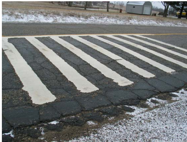
Figure 3.1. Raised-paint rumble strips
