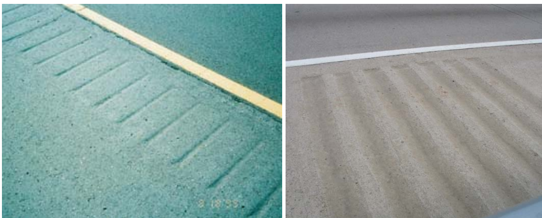
Figure 3.2. Rolled-in rumble strips (on the right: an intermittent type on concrete)
