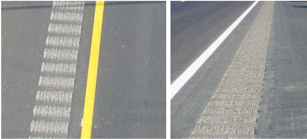
Figure 3.3. Milled-in rumble strips
