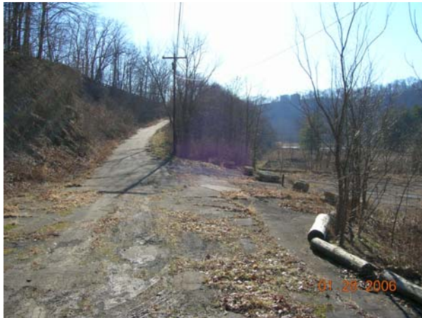
Figure 4.5 Degraded entry drive. Stormwater from culverts at the top of the hill continue to erode the entry hardscape.
