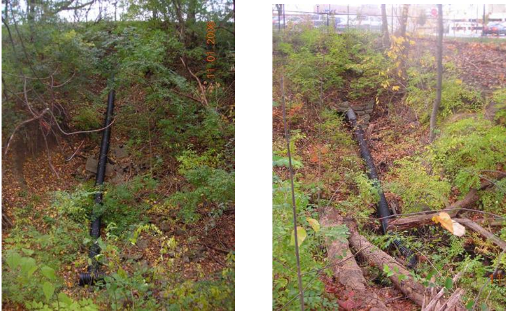
Figure 4.6 Erosion prevention solution for southeastern slope. The black pipes allow for the concentrated discharge to be directed towards the bottom of the slope, preventing erosion. (photographs from School Girl's Glen, Ann Arbor, MI).
