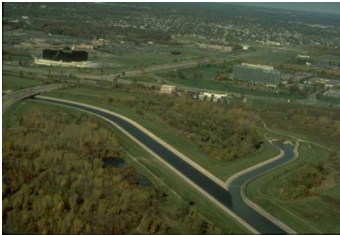
Figure 3.4: Rouge River’s concrete channel closely resembles the existing condition of the Flint River ( http://www.miseagrant.umich.edu/greenways/08LGa.html ).
