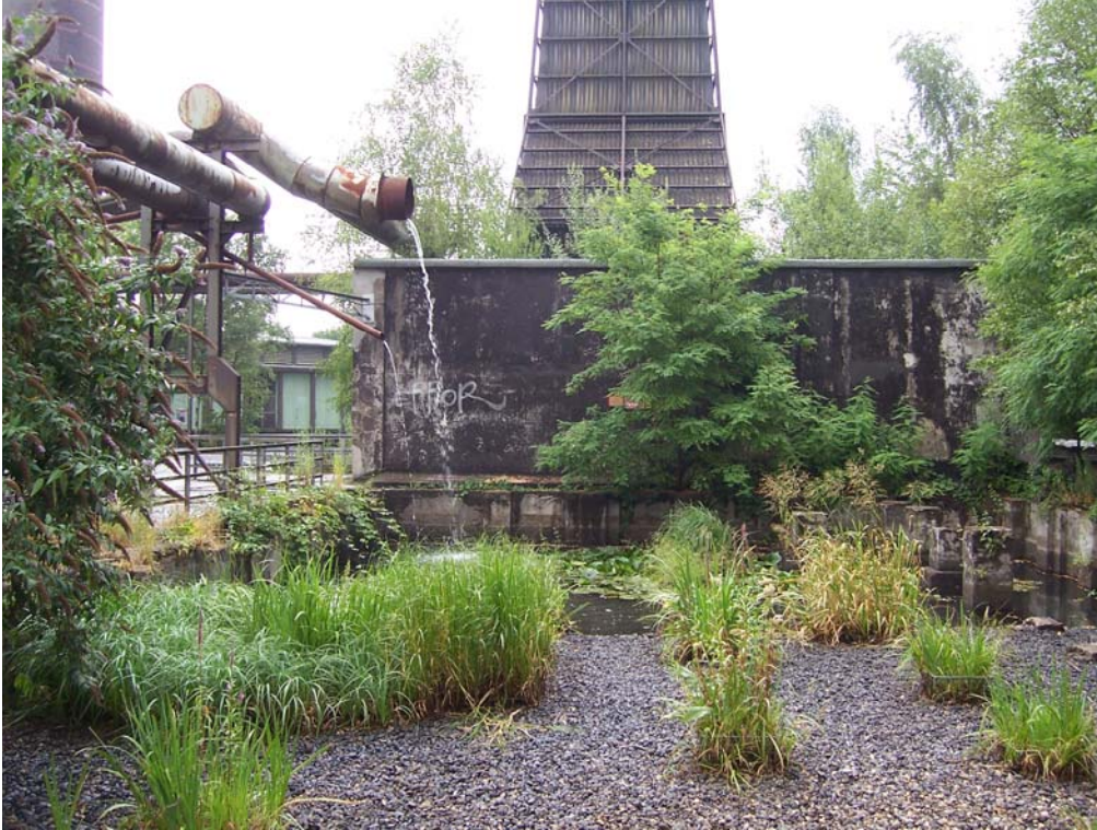
Figure 3.15: Reuse of overhead pipes carries clean rain water into this garden where it is detained and infiltrated into clean soils (Emily Marshall).
