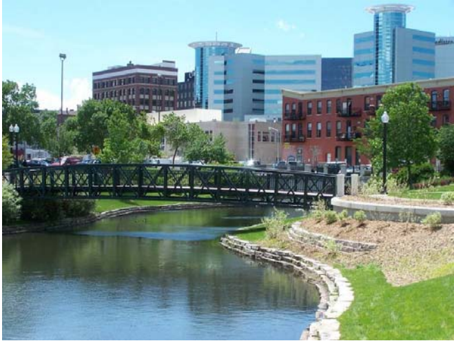
Figure 5.8: River terraces were created when Arcadia Creek was daylighted and restored in Kalamazoo, MI ( www.city-data.com/city/Kalamazoo-Michigan ).
