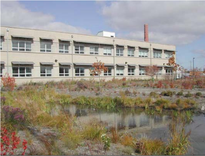
Figure 3.18: Stormwater wetland, installed in clean soil brought on site to replace slag heap (CCGT).
