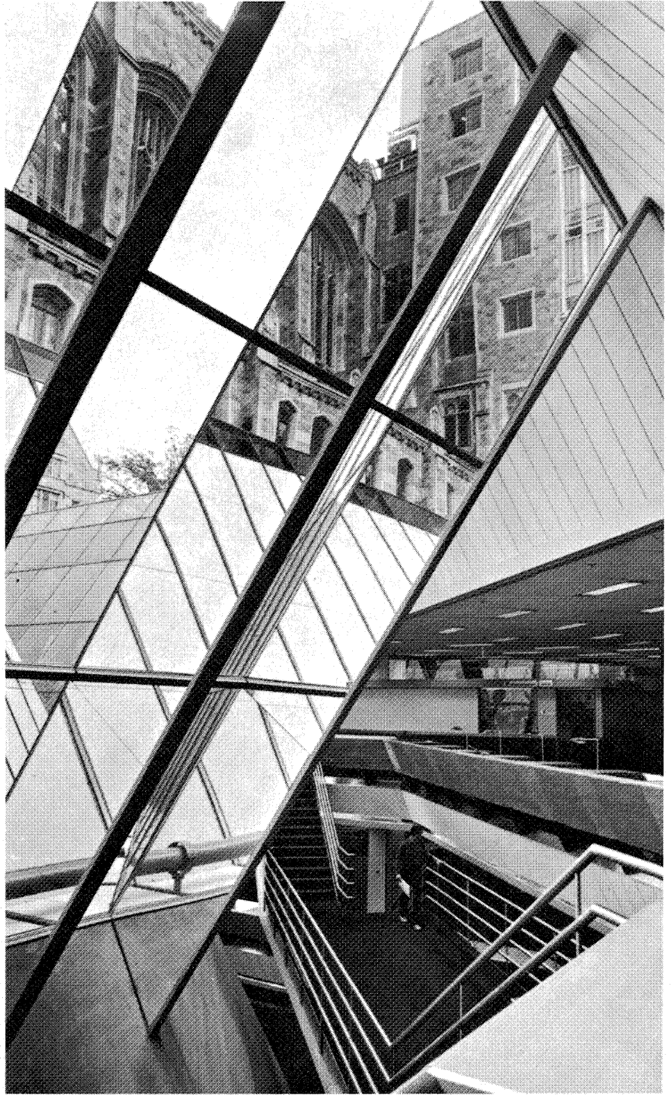
The new law library is illuminated by an enormous lightwell which furnishes light to all three underground floors. (Photo by Kim Hill)
