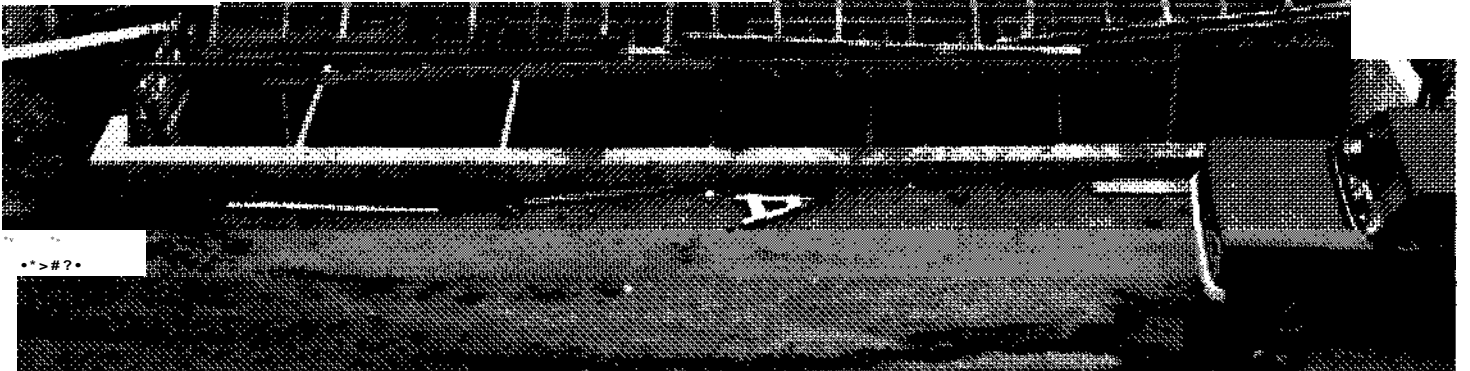
No, this is not a waffle iron. It is the plywood base and fiber glas domes for the first floor concrete slab under the new library. The "waffle" appearance of the floor underside will be the ceilings for the library, classrooms, and office areas.
