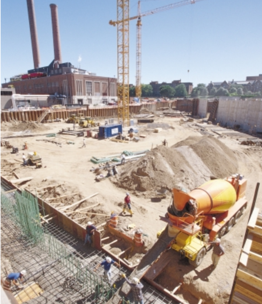
Construction has begun on the University's $100 million Life Sciences Institute.
