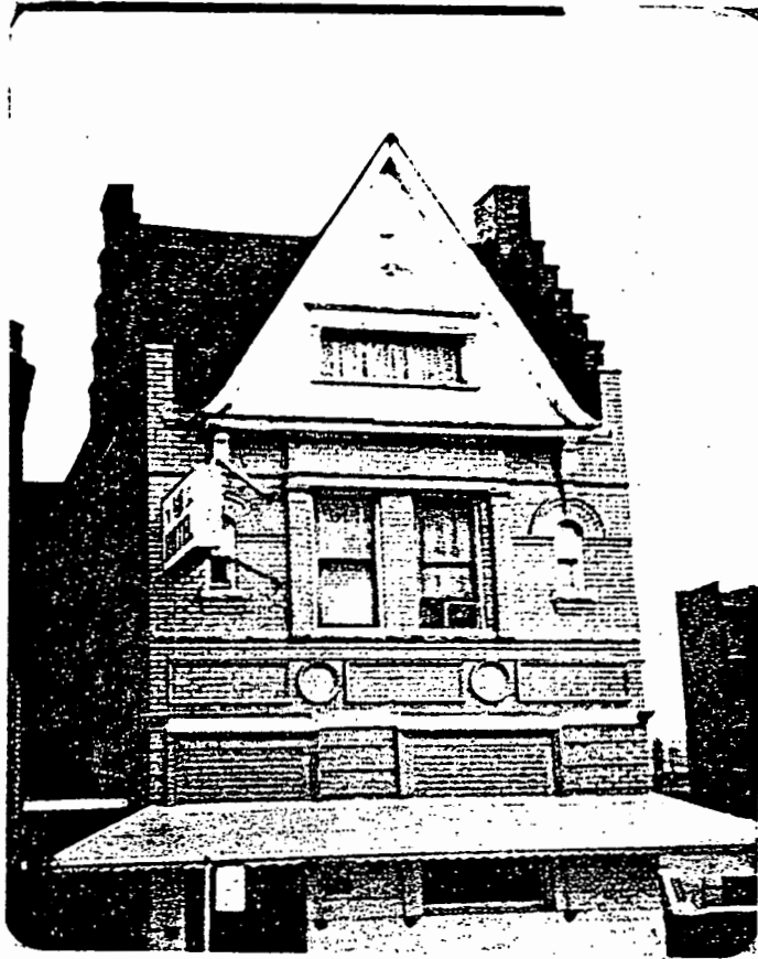
448 Montcalm (146 before 1920); a building in the German style built before 1889.
