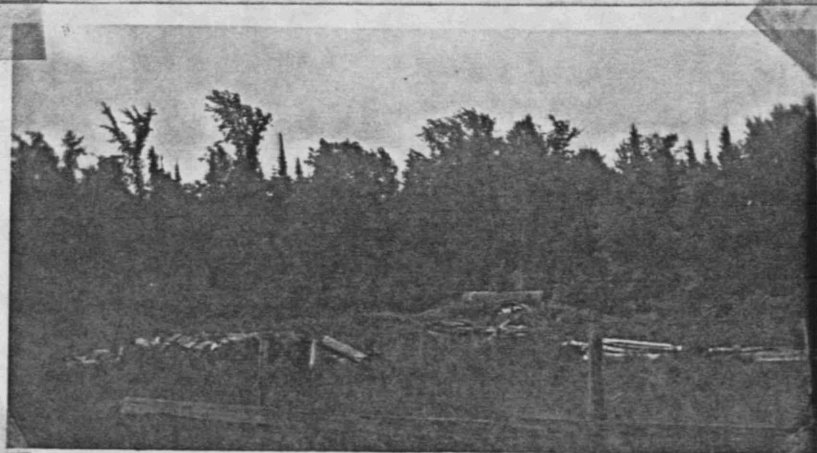
Fig. 3. Sawmill entrance at northeastern part of Bog Ditto
