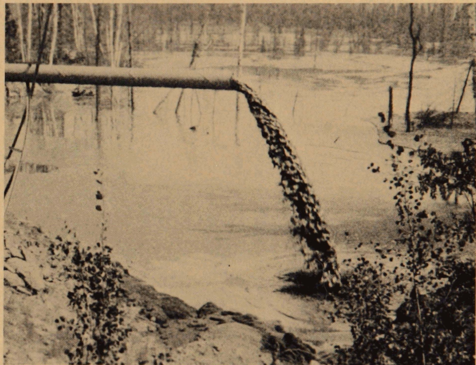
Iron tailings discharge pipe at mine near Ishpeming, Michigan.
