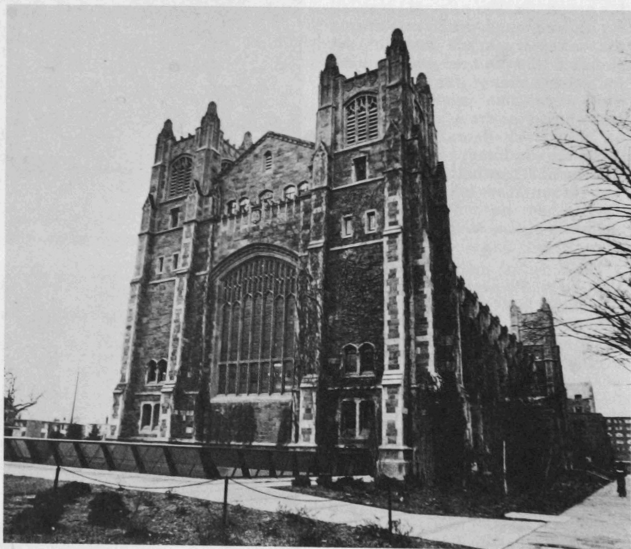
The east end of the Legal Research Library with the new addition in the (literal) foreground.
