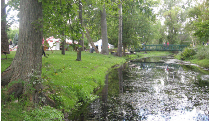
Eroding banks of Millrace new bridge in background (Photo by S. Mattke-Robinson)
