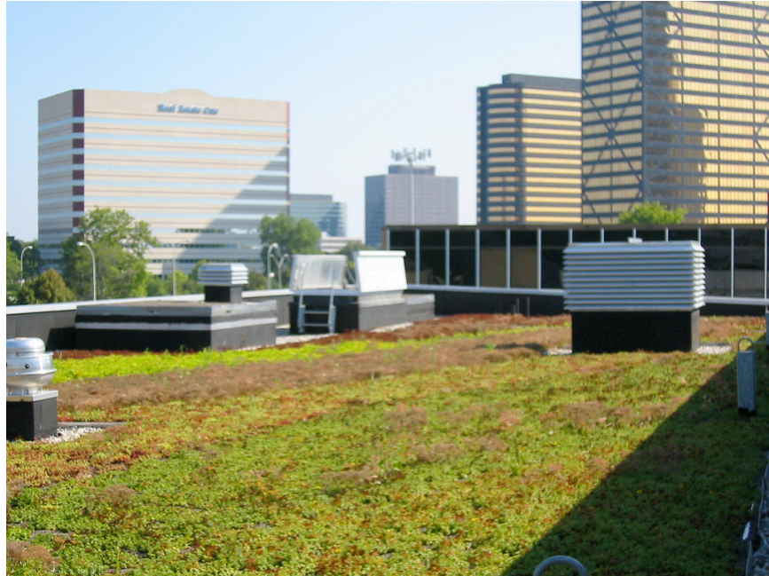
Figure 2.5 Extensive green roof at Lawrence Technological University in Southfield, Michigan (photograph by author).
