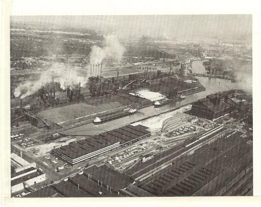
Aerial view of the Ford Motor Company complex, steel mill, and auto assembly plants at River Rouge, Michigan. The Ford Motor Company's River Rouge industrial complex near Detroit, Michigan, is a vertically integrated system in which basic raw materials, including iron ore, limestone, and coal, are used to produce steel which, within a few days, is incorporated into the engines, frames, bodies, and parts of completed automobiles. (Photo courtesy of the Ford Motor Company)
