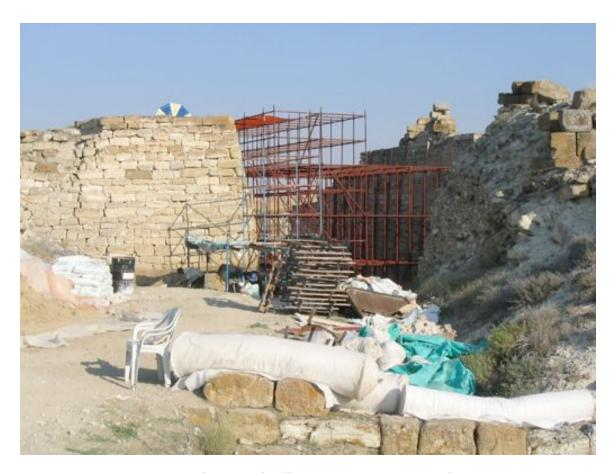
Figure 7-4. The citadel gate, Gordion. Scaffolding allows injection of hydraulic lime into the structure (D. Shoup)
