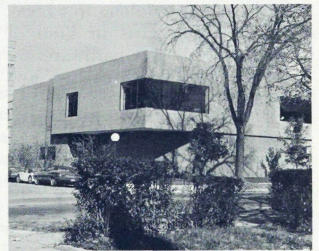
CLAYTON G. HALE AUDITORIUM —A 500-seat hall and facilities for conferences and teaching make up this two-story structure named for major donor Clayton G. Hale. It is separate from but connected to the main Business Administration building.
