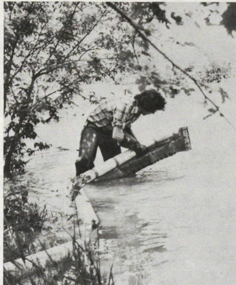
Mark Torf sets an oil containment boom across a creek to trap a spill which can then be pumped from the surface of the water.
