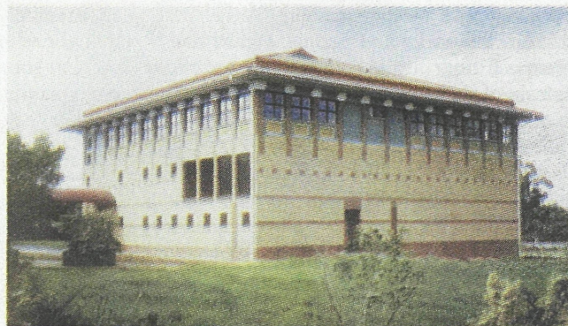
Center for Cultural Studies Building, University of Fort Hare.
