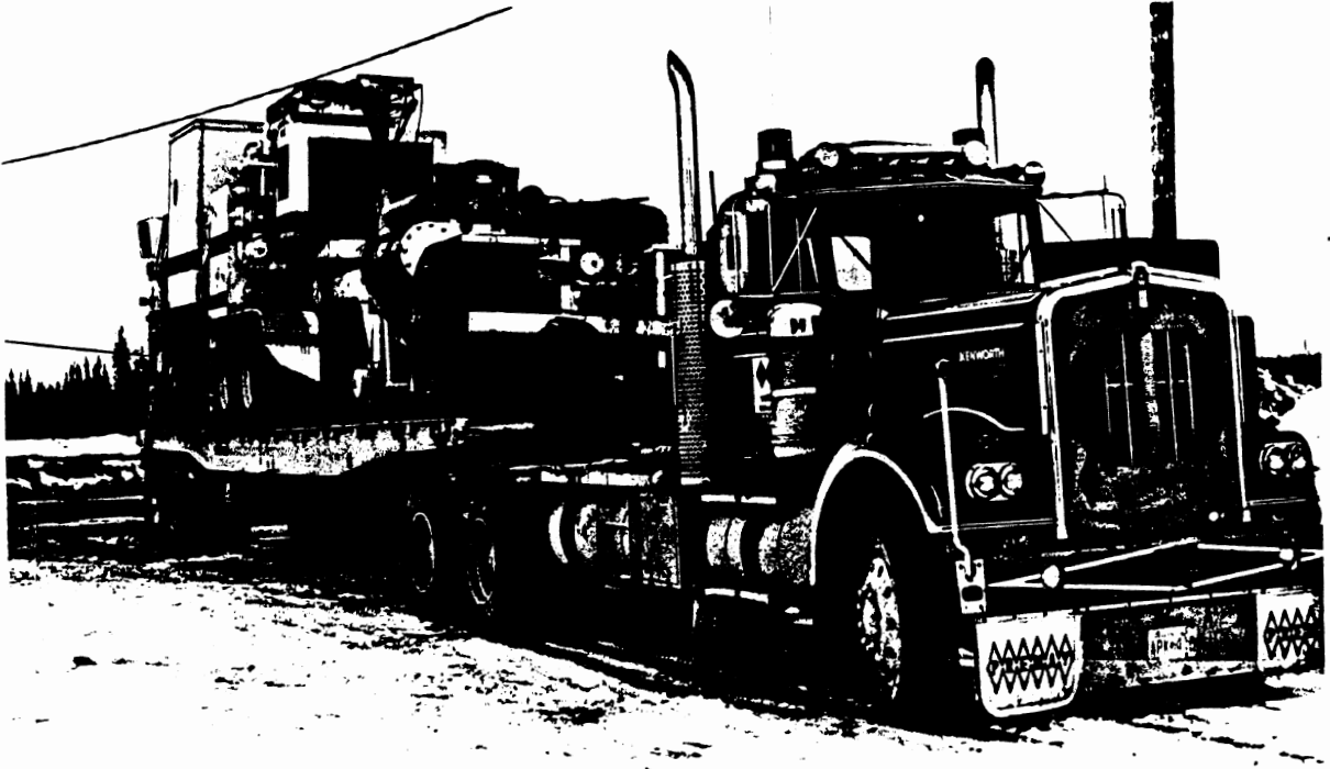
Figure 3 Mobile Dynamometer on hauler for trip to Lake Wollaston
