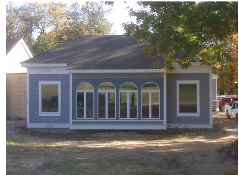
Helga House: View from West
