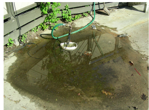
Wastewater in Golf Maintenance Area
