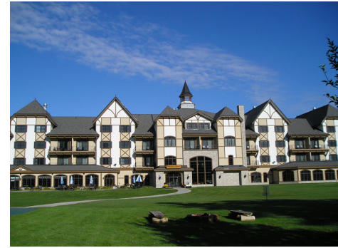
Mountain Grand Lodge: View from West
