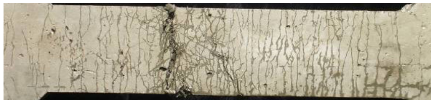
Cracking spacing and pattern of Torex fiber 2% reinforced specimen
