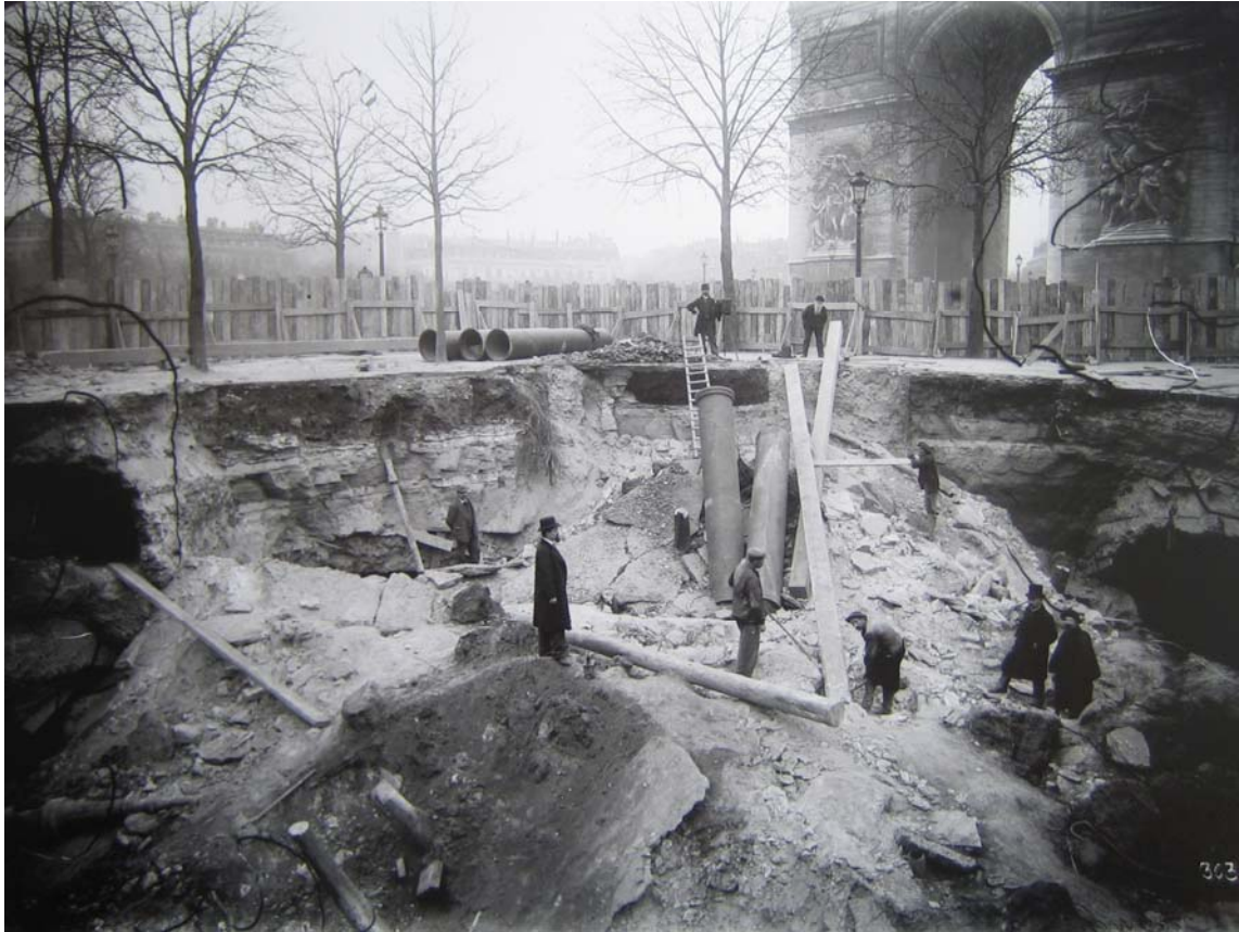
Figure 16: The Arc de Triomphe overlooks a chaotic scene. A Métro tunnel in progress under the place de l'Étoile collapsed on December 11, 1899. Here, workers and engineers survey the damage. The two figures standing on the rim at the back of the photograph are members of the photographic crew that took the picture. 112
