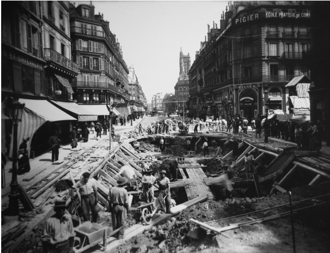
Figure 15: The rue de Rivoli, June 30, 1899 (looking east toward the Hôtel de Ville). In the foreground, workers are building the vaulted ceiling of the station at Châtelet, the final step before relaying the road surface. One can see how little of the street is left open on either side of the construction site. 108
