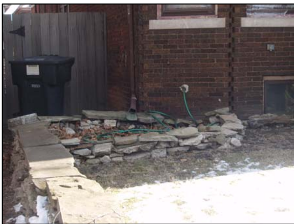
Figure 16. Rain garden on Avery Street. Photo by L. Miller
