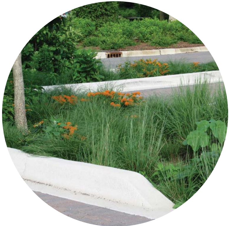
I 14. Parking Lot Bioretention Chicago, IL
