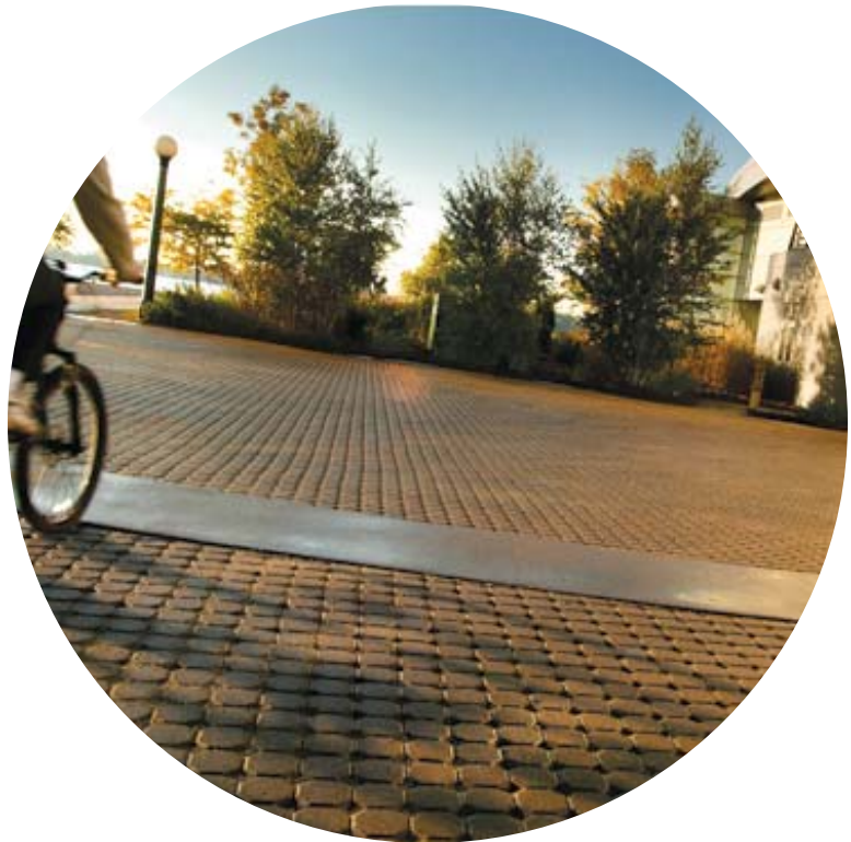
108. Permeable Pavement Street Unilock
