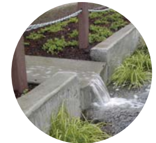
158. Runnel downspout into raingarden Portland, OR
