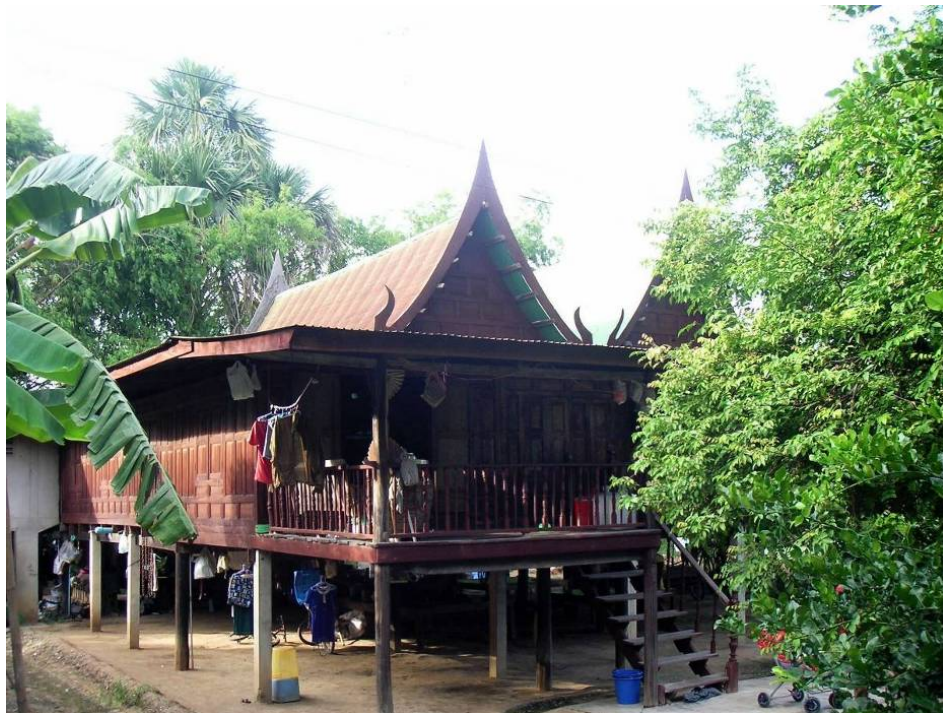
Figure 63: A modified farmer's home with a single access stairway to the upper platform
