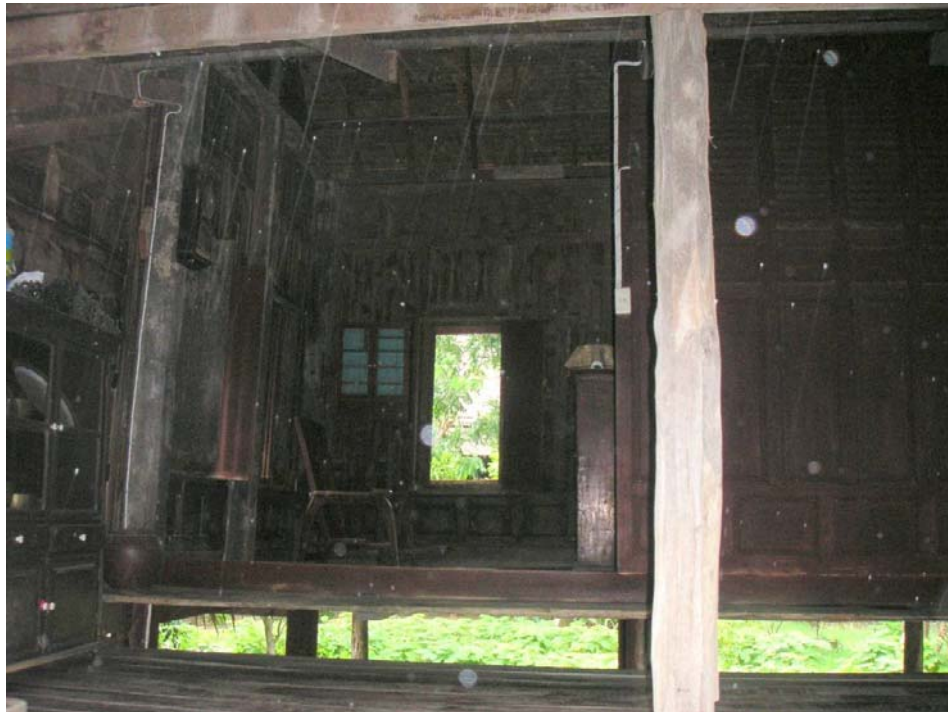
Figure 52: Floor gap between the verandah and the living compartment that is large enough for a person to crawl into the house
