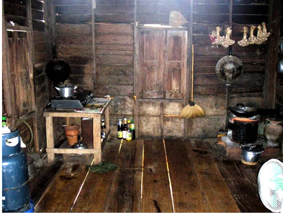
Figure 71: Increasing use of solid wall panels results in inefficient air ventilation in a modified kitchen and the whole dwelling unit
