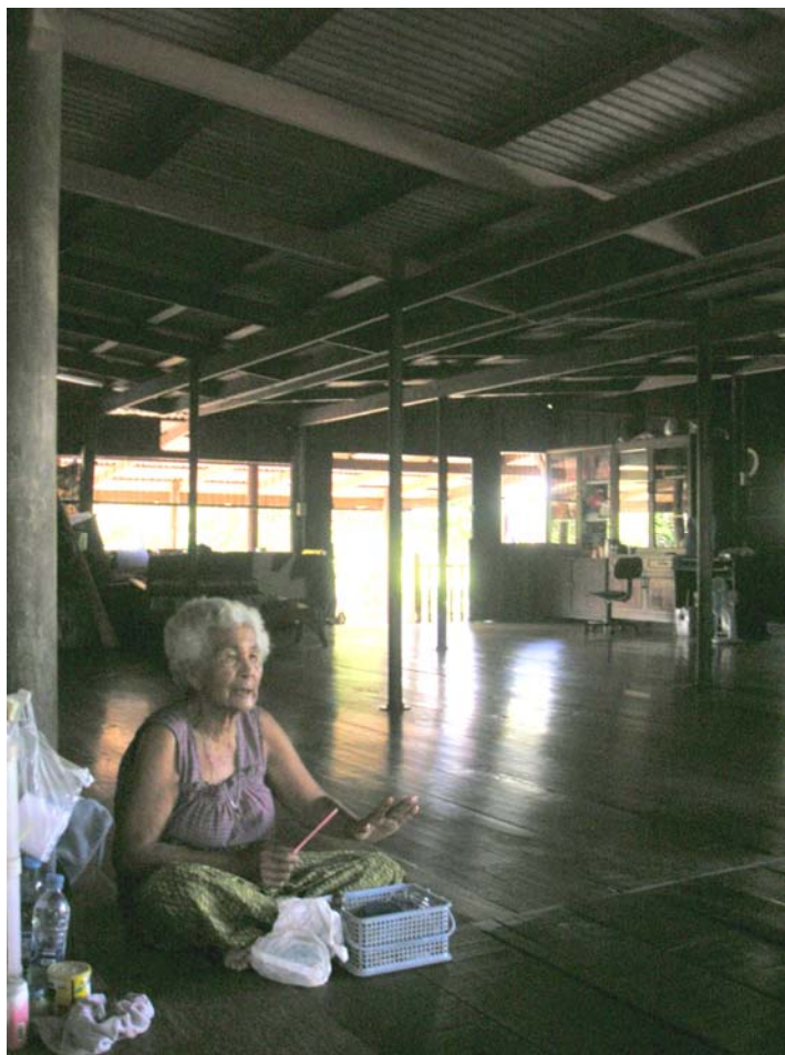
Figure 80: The multipurpose hall has been converted from combining the terrace and the verandah under the newly built roof that extended from the eaves of the original compartment
