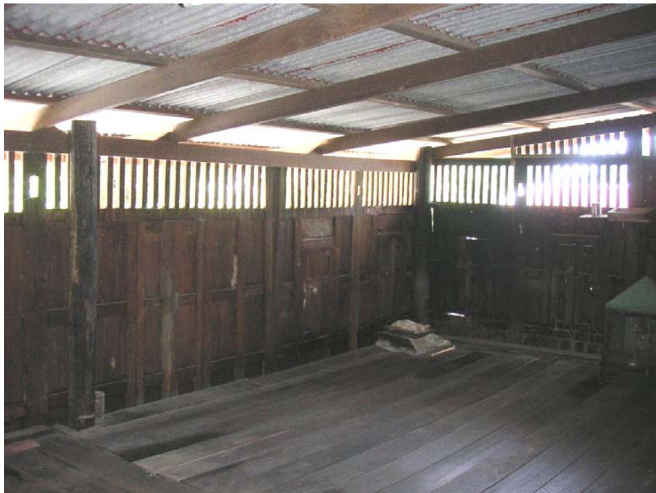
Figure 100: The foldable wall surrounding the terrace is now permanently closed
