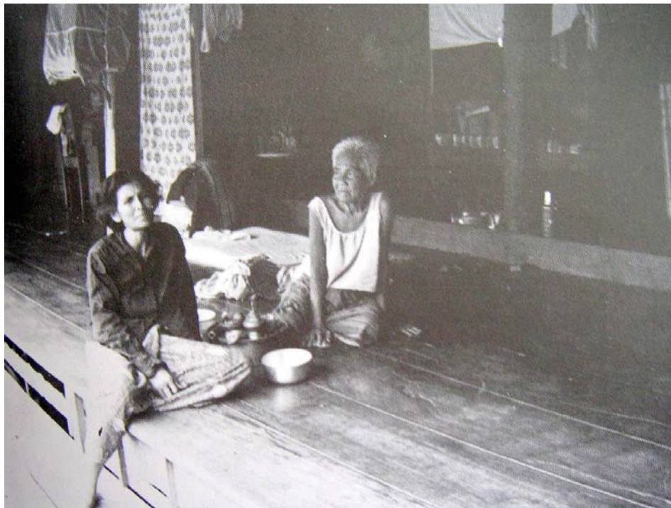
Figure 65: The different flooring level between the terrace and the verandah that serves as a seating area
