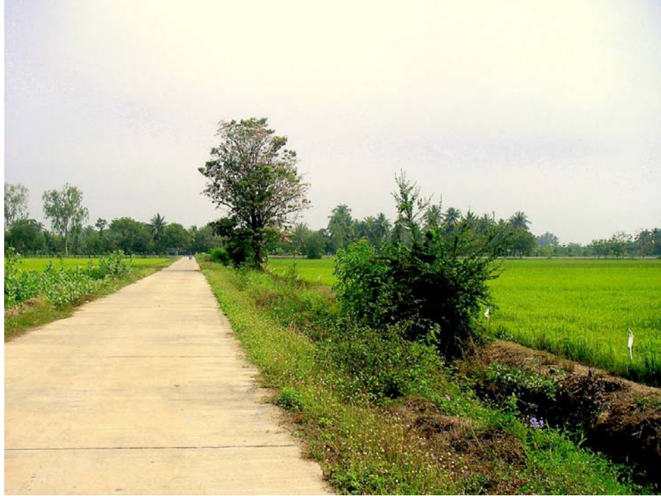
Figure 12: Concrete paved roadway provides easy access to today's paddy field
