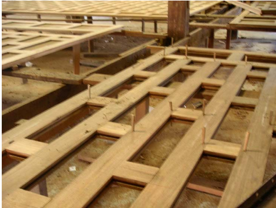
Figure 47: One of several types of wall panels waiting to be assembled in the master builder's shop
