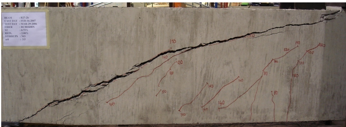
Fig. 4-125: Crack pattern after failure – Beam B27-2b
