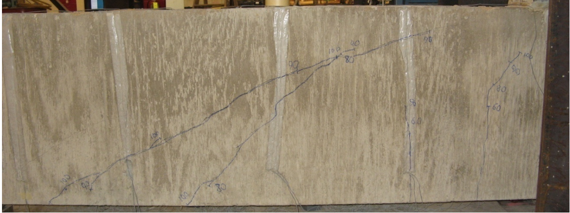
Fig. 4-190: Crack pattern prior to failure – Beam B27-8
