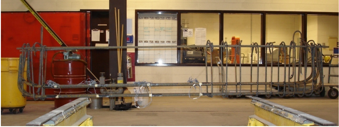
(a) Reinforcing cage ready for placement
