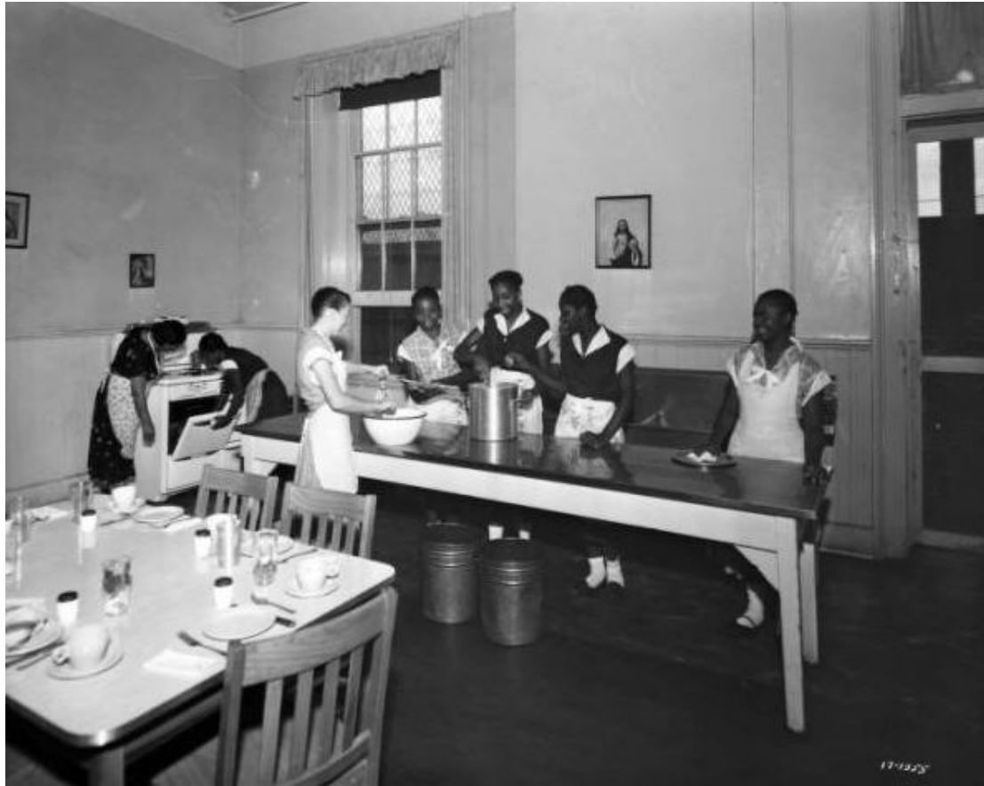
Figure 4.7 Convent of the Good Shepherd Kitchen, 1955 (Courtesy of The Historic New Orleans Collection)
