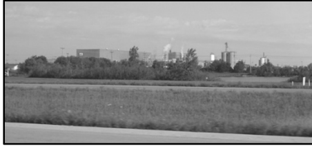
Figure 3.2: Frito Lay plant east of Frankfort on SR 28
