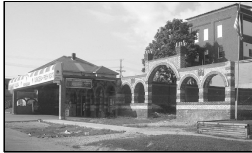
Figure 3.5: Mexican grocery with masonry wall
