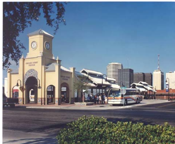
The Staples Street Station in Corpus Christi.
