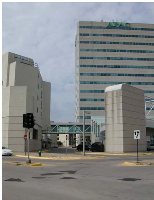
Entrance to intercity bus station adjacent to GTC/APAC.
