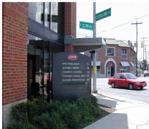
Signage showing the occupants of the Linden Transit Center, with the Linden Café across the street.
