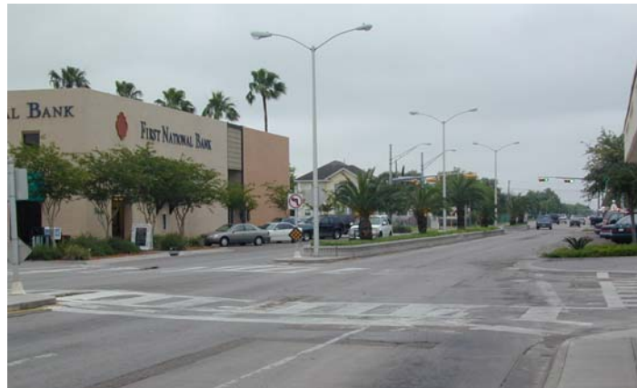
Landscaping, lighting, and pedestrian improvements near the Six Points Station funded through the Livable Communities Initiative Grant.
