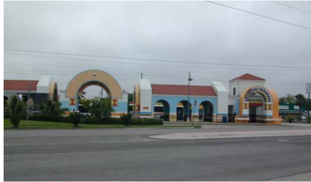
The Port Ayres Station reflects the colorful nature of CCRTA's stations.
