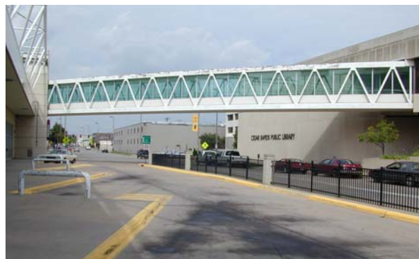
An example of an enclosed pedestrian skywalk connecting the GTC and the Cedar Rapids Public Library.
