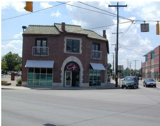
The Linden Café building that also hosts a barber shop and offices located directly across the street from the Linden Transit Center.
