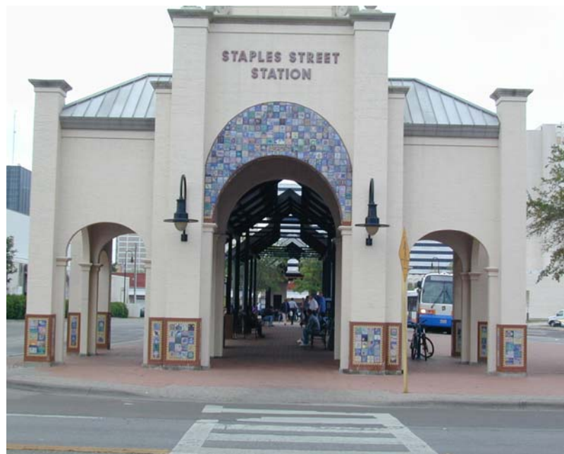
View of the Staples Street Station looking through the facility from the head house.
