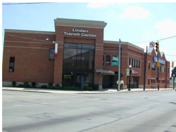
The Linden Transit Center located at the intersection of Cleveland and 11 th Avenues.
