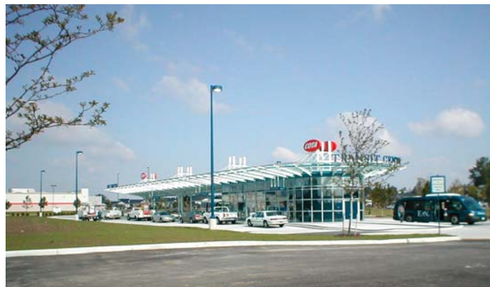
A contemporary example of a Bus Transfer Center.
