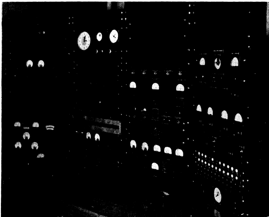
Fig. 4. A view of the control panel.
