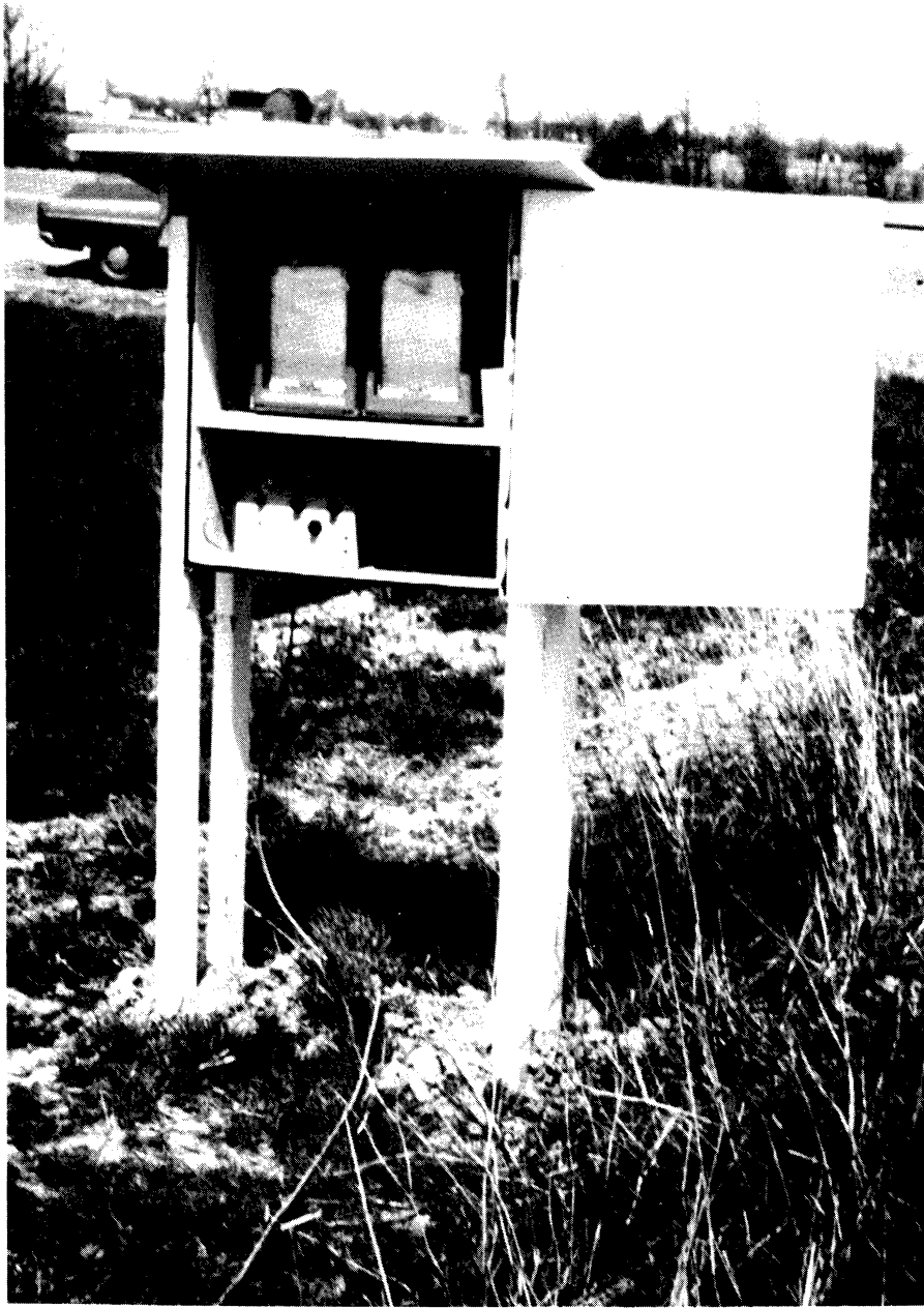
Figure 4. Shelter containing wind translator, recorders, and battery
