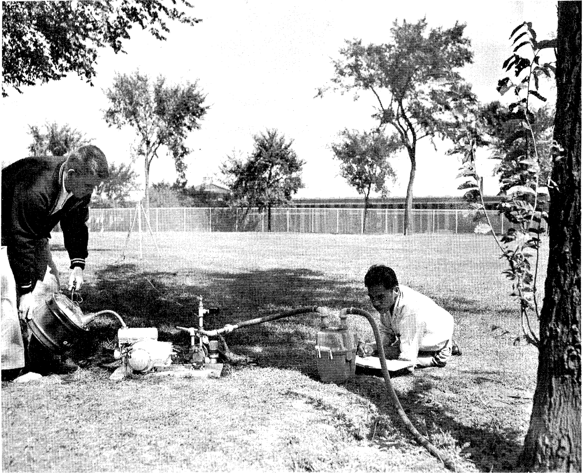
Fig. 3.11. Portable volumetric pollen sampler showing gasoline motor, dry test meter, and in the background tripod supporting sampler.
