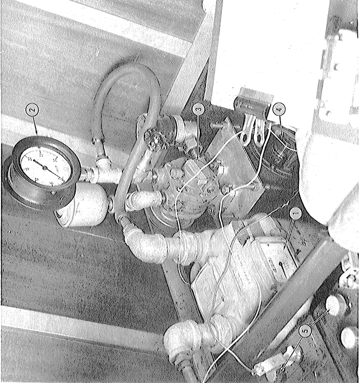
Fig. 32. Interior-mounted equipment, aerial sampling program.
