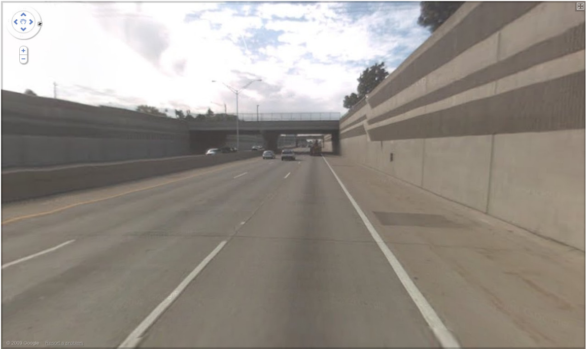
Figure 4-5 Arterials with limited access: Interstate 696, Michigan
