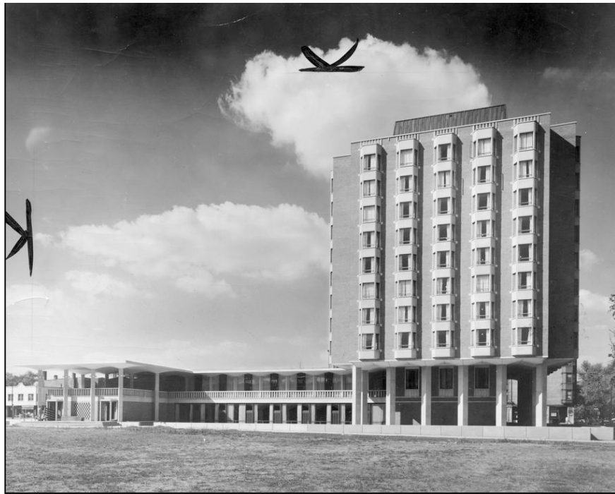
Figure 4.9. Pierce Hall, designed by Harry Weese & Associates, viewed from the south (within the campus). Two-story lounges in the tower have rendered interior the social and leisure space that formerly was distributed throughout the block and accessed by entry on E. 55 th St. The density and diversity on the block has been transformed into an unchangeable, uniform set of uses and users. (Buildings and Grounds Photographs. UCSC).
