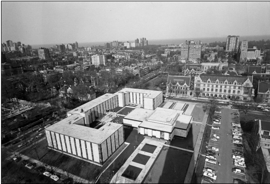
Fig 4.5. Aerial view of Woodward Court looking east-northeast towards the lake. E. 58 th St. runs east-west to the north of the dormitory. The dining hall creates the fourth side of the quadrangle and helps govern the pedestrian activity of residents and visitors, channeling them directly east to the Laboratory Schools and west to Rockefeller Chapel. (UCSC)
