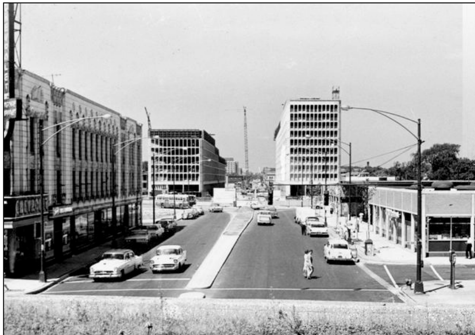
Fig 4.13. Hyde Park viewed from the same spot during redevelopment. East 55 th has been widened and routed around the University Park condominium towers, under construction in the photo, designed by I.M. Pei and Associates. Buildings on north side of East 55 th have been demolished and redeveloped as part of Hyde Park A Project. (Buildings and Grounds Photographs. UCSC).
