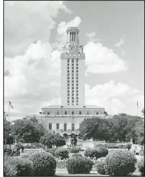
Fig 3.8. Main Building with Littlefield Fountain in background, UT-Austin. (CAHUT)
