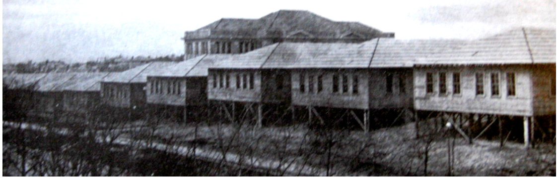
Fig 3.2. The UT Shacks. Built in the World War I era, these structures remained in use until the middle 1930s. (CAHUT)
