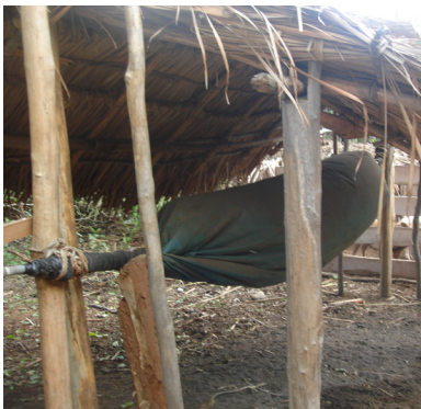
Figure 46. This expandable bag within the biodigester system holds the generated methane before it is burned. Photo credit: P. Liao
