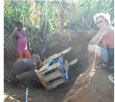
Figure 62. Ho Avy fixing the treadle pump. Photo credit: O. Lau
