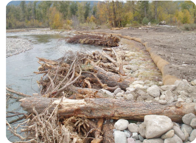
Fig. 26: An engineered log jam slows erosion along riverbanks.
