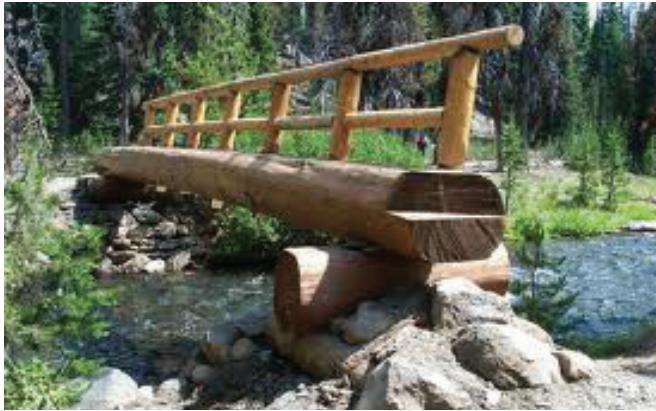
Fig. 61: Single-log stringer bridge
