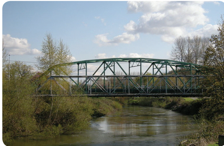
Meeker St. Bridge in Kent, WA (photo credit: Joe Mable)
