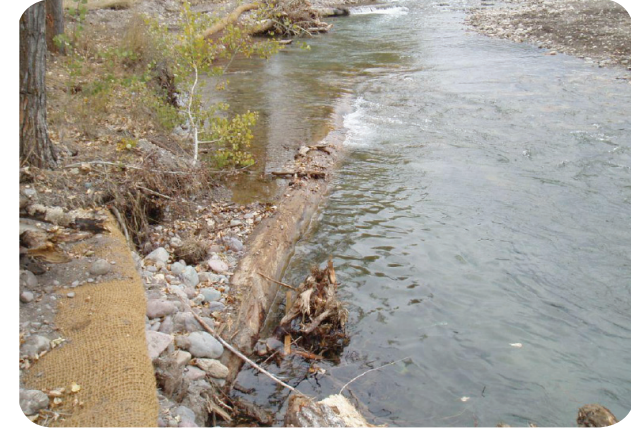
Fig. 25: A straight vein redirects current to the center of the channel to prevent erosion.
