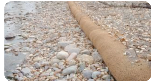
Fig. 27: A coir log is a bioengineering structure used for bank stabilization.
