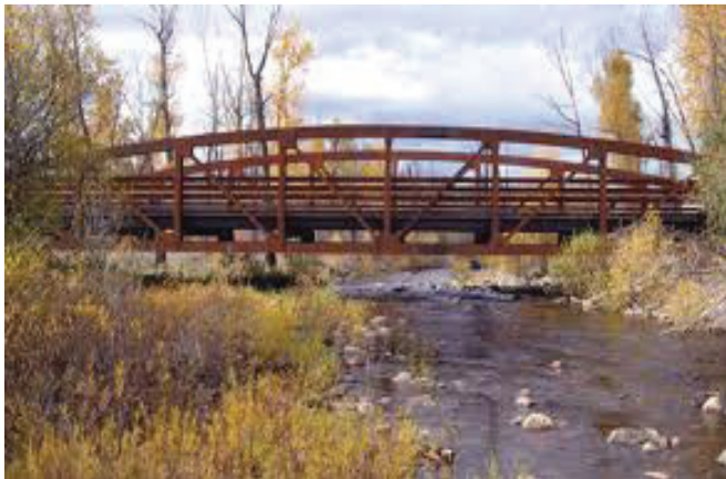
Fig. 65: Steel truss bridge
