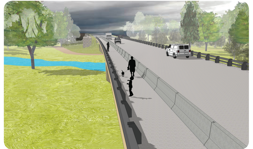
Fig. 2.20 Looking south across the bridge. The pedestrian lane is approximately 8' wide.
