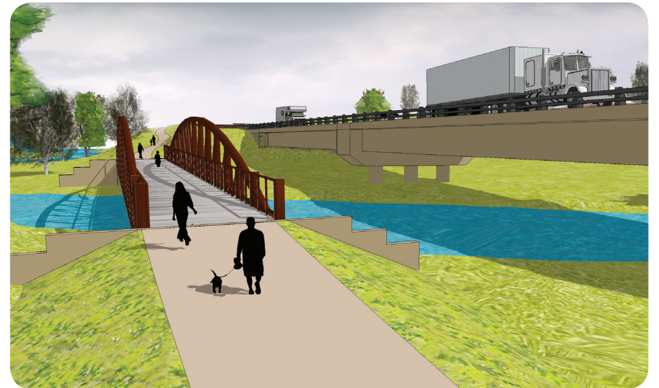
Fig. 2.14: Looking north at the pedestrian bridge. This style of bridge is known as a steel truss construction.
