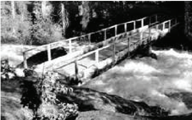
Fig. 63: Multiple-log stringer bridge
