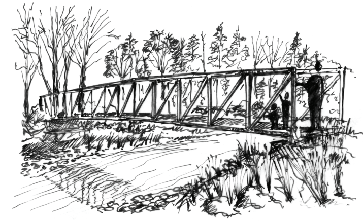
Fig. 66: Steel truss bridge
