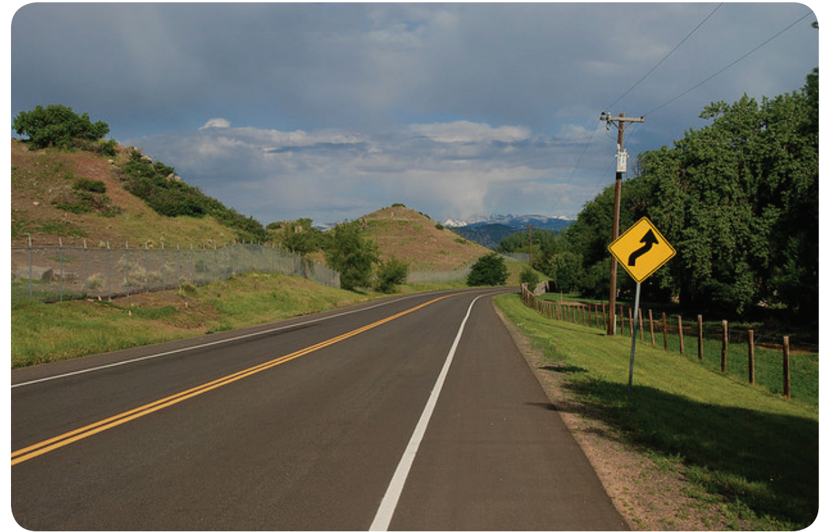
Fig. 3.5: A shoulder bikeway outside of Boulder, Colorado (photo credit: Let Ideas Compete).
