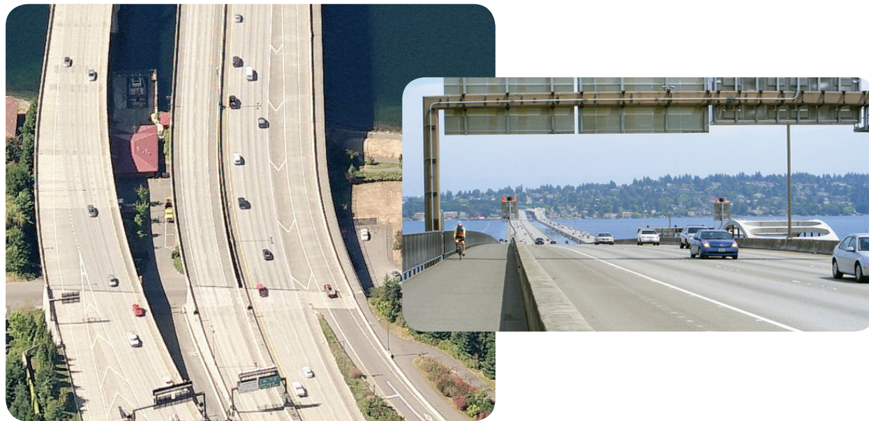
I-90 bridge over Lake Washington, Seattle, WA. (Large photo: Bing Maps, copyright Microsoft 2011. Inset: flickr.com)
