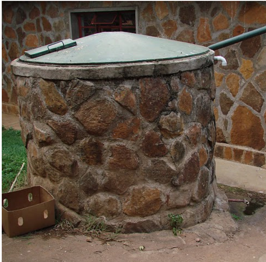
Image W-i 11: plumbing set-up for small water tank by kitchen. Photograph by Melissa Antokal, 7 August 2010.
