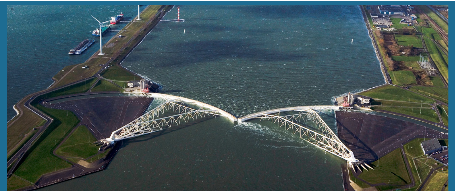
Figure 121: Innovative sea barriers to protect against storm surge and sea level rise
