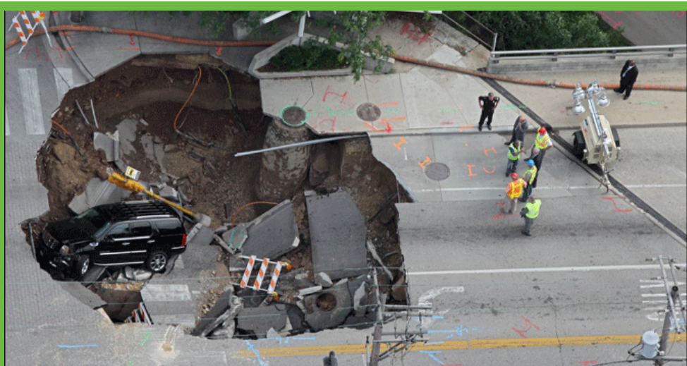
Figure 96: Sink hole created by the July 22nd Milwaukee flood
