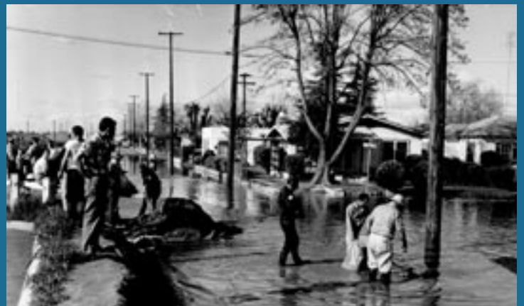
Figure 9: Flooding in Fresno County on March 23, 1958
