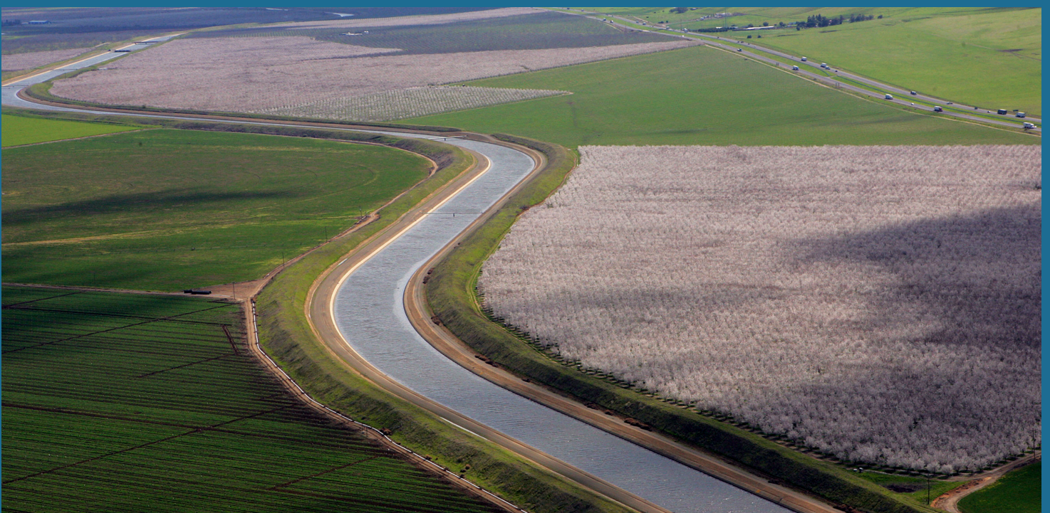
Figure 117: Proper management of water is essential to the quality of life in California
