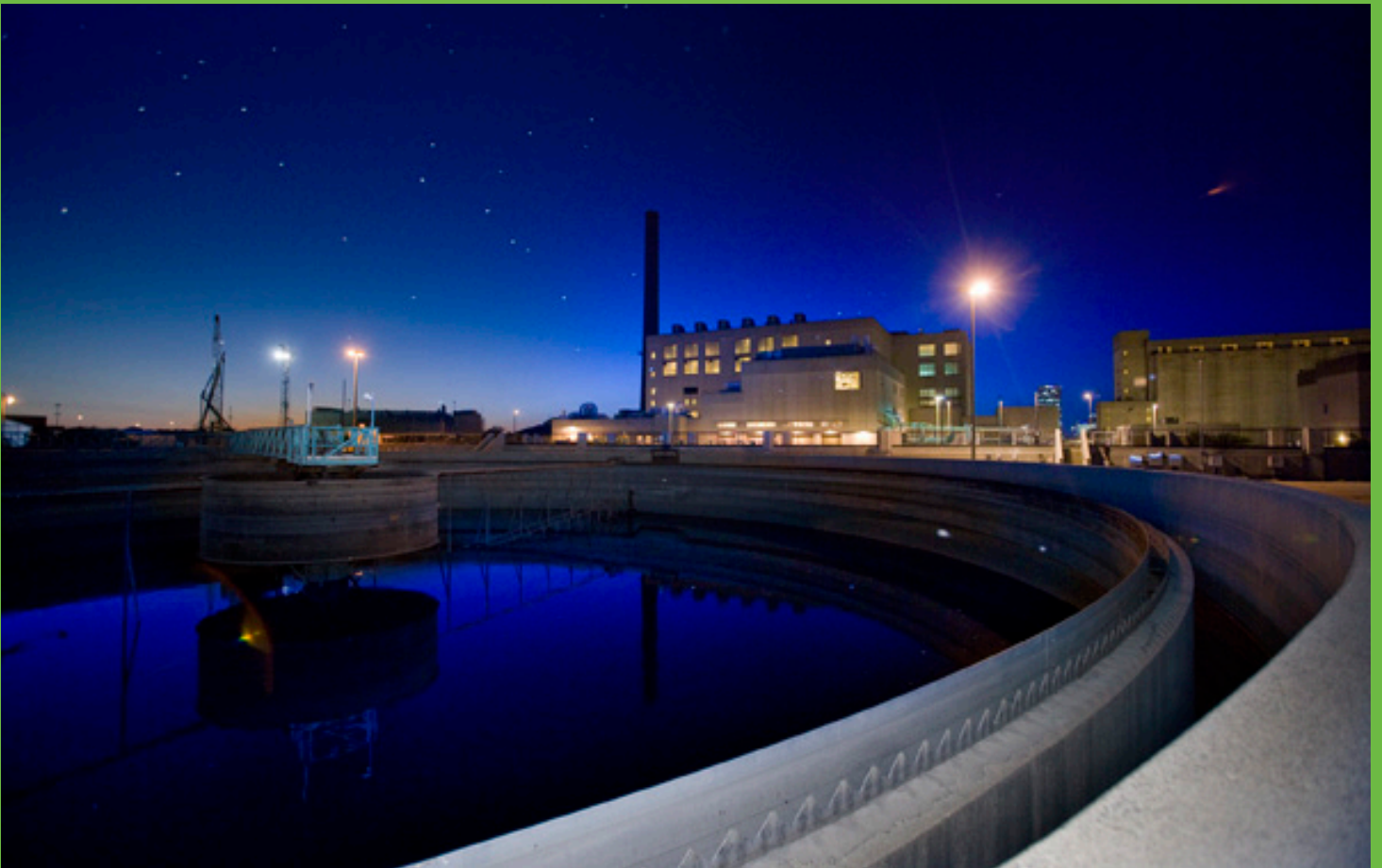
Figure 94: Milwaukee Wastewater Treatment Plant at night
