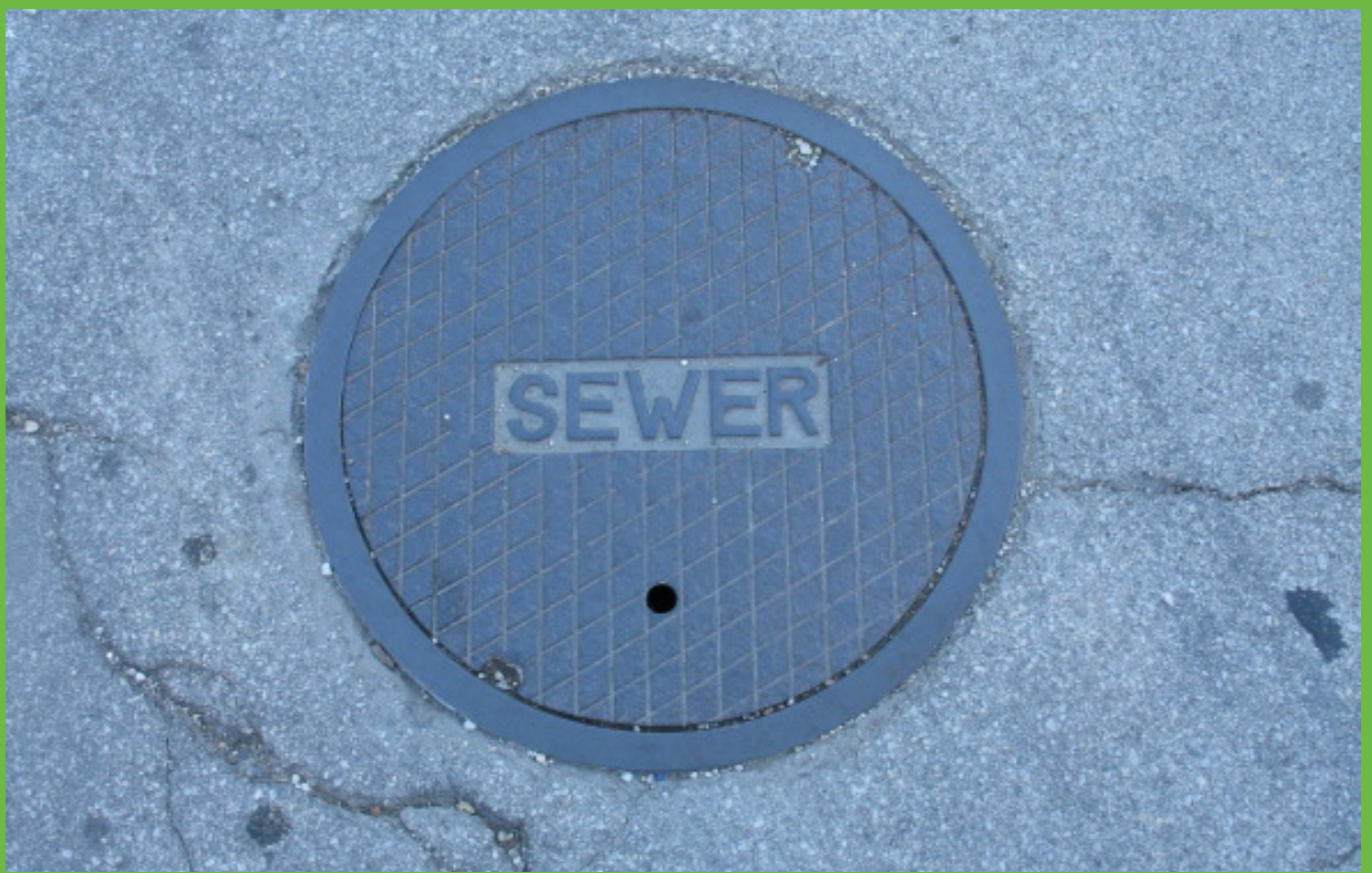
Figure 104: Milwaukee has a combined sanitary and storm water sewer system which historically has had overflow problems
