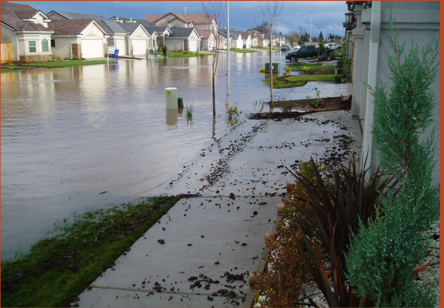
Figure 61: Insufficient suburban stormwater infrastructure lead to massive flooding in Fresno on January 2nd, 2006
