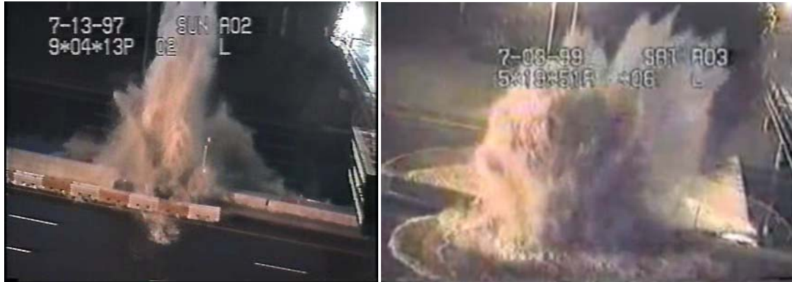
Figure 2.1: Geyser events in the I-35W storm sewer tunnel of Minneapolis, Minnesota
