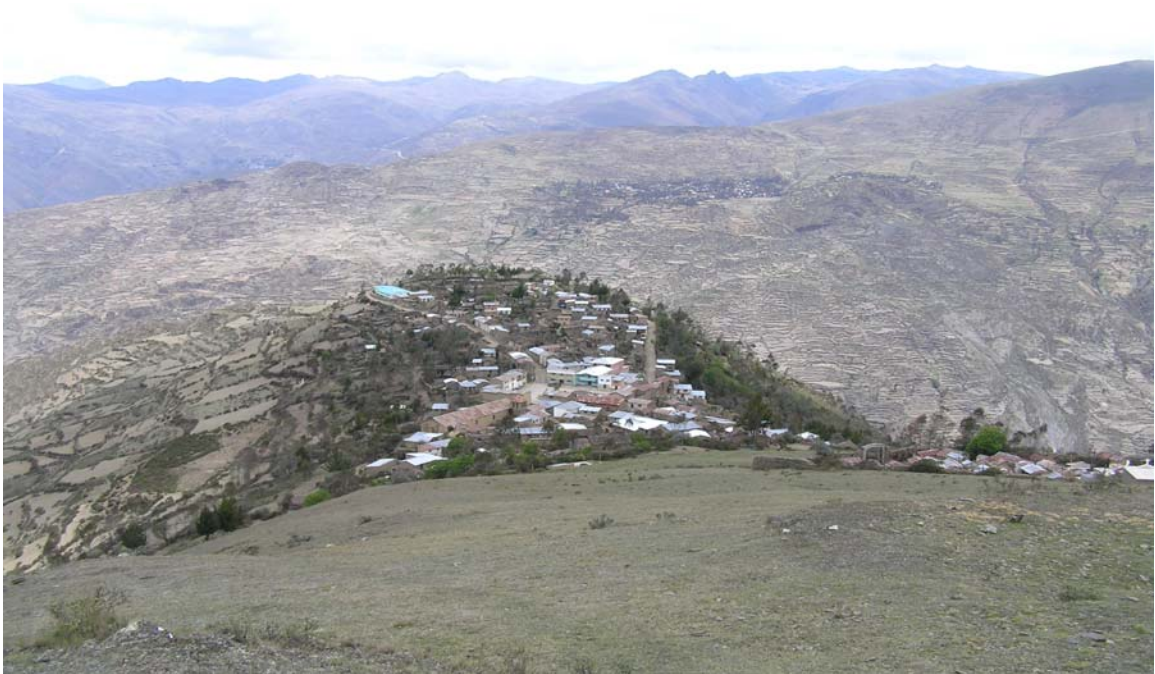
Figure 4: An aerial view of Curva.
