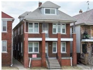
Exterior: brick, type: two-family flat
