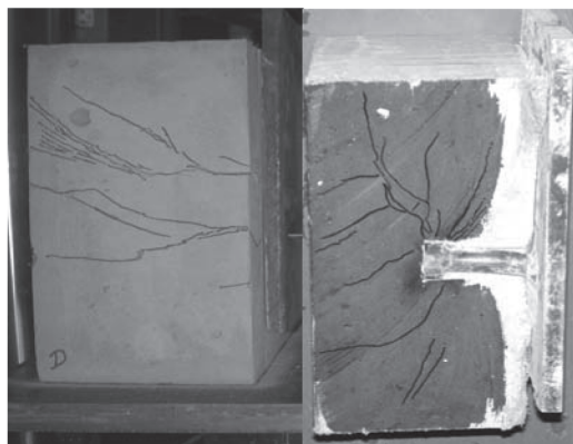
Figure 7. Microcracks developed outside (left) and inside (right, cut section along shear stud) of ECC specimen
