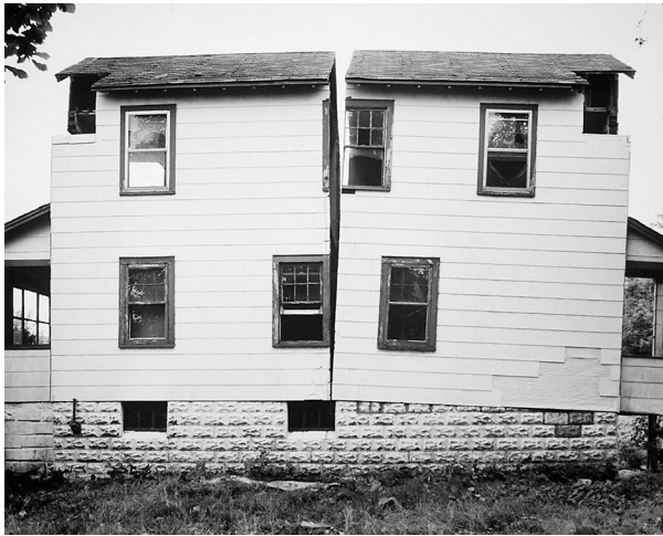
9. Gordon Matta-Clark, Splitting (exterior), 1973
