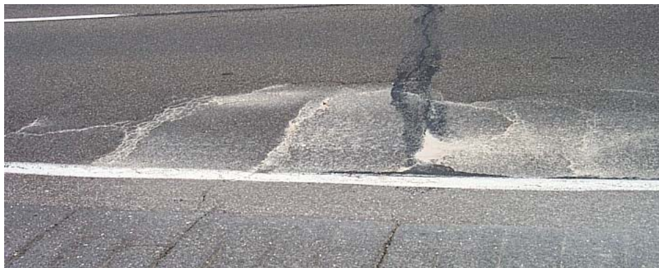
Figure 30. A fatigued area with pumping on section 0661 in august 2000.
