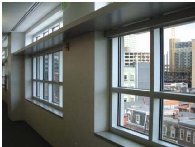
Fig. 13: Interior Light Shelves [24]
