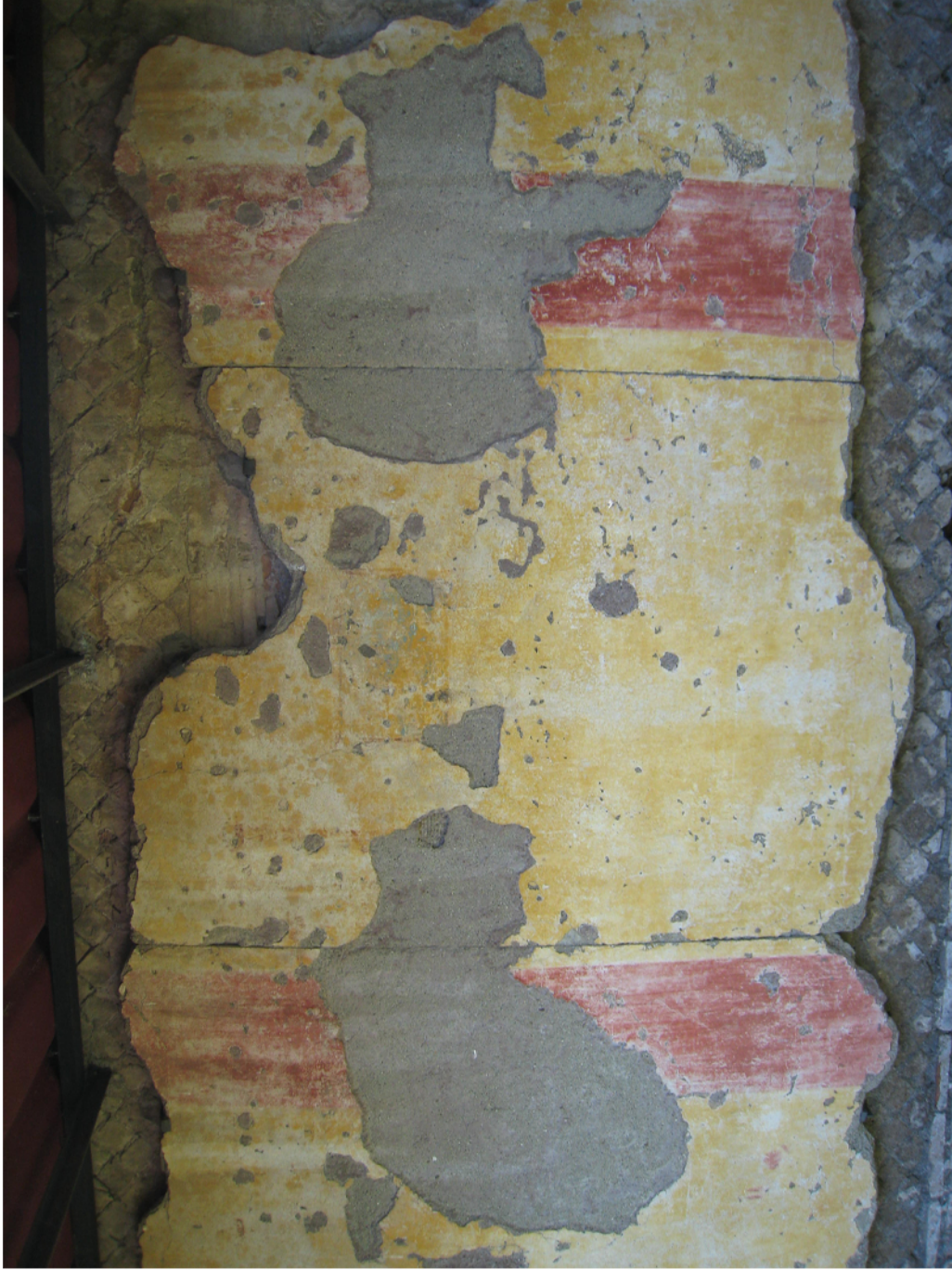
Fig. 53. Apartment III, IX, 16, room 6. View of east wall. (KAR 2009)
