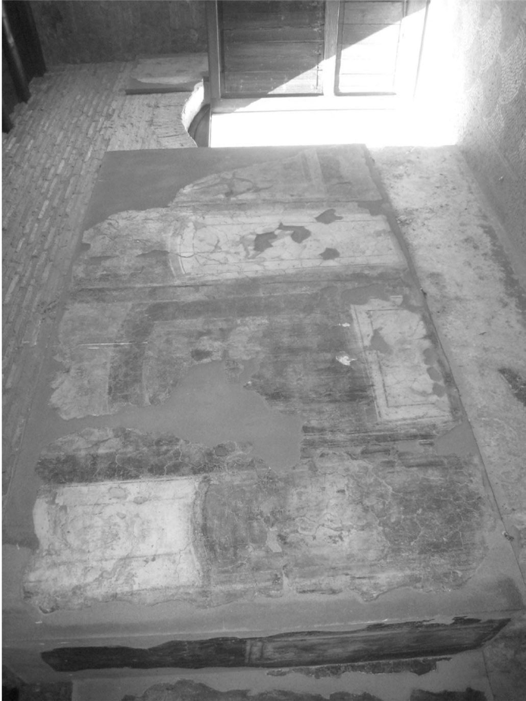
Fig. 42. Inn of the Peacock, room 6. View of north wall with panel system of painted decoration on a polychrome background. (KAR 2009)
