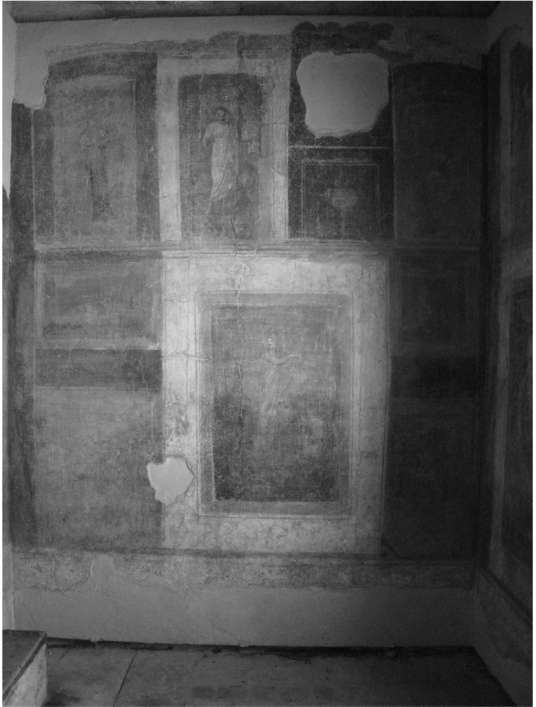
Fig. 41. Inn of the Peacock, room 9. View of north wall with panel system of painted decoration on a polychrome background. (KAR 2009)
