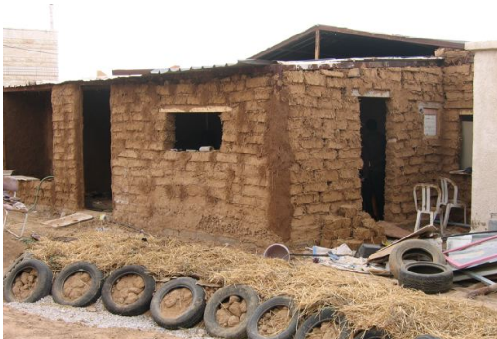
Image 6: Mufid Abu Assa's permaculture house, under construction.
