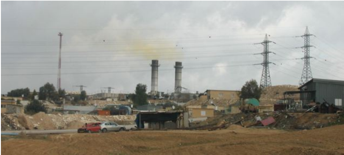
Image 15: One side of Wadi al-Na'am, next to the electricity plant.
